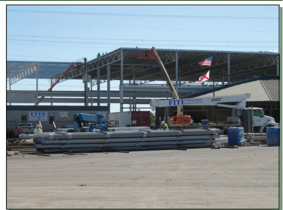
Rebuilding is underway at Independence Tube
